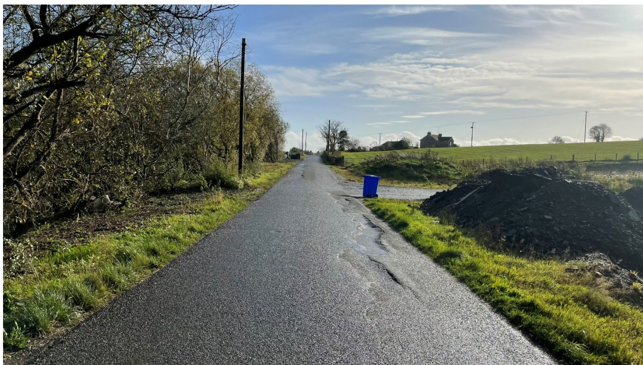
Figure 5.1 – Existing Road Condition on Cavan Road
